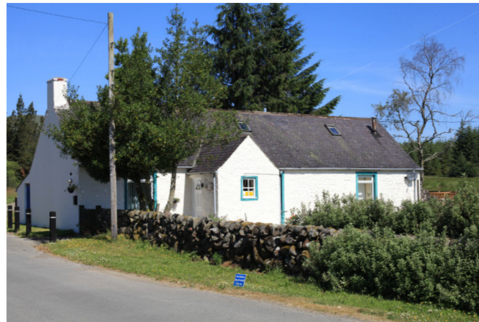
South-eastern elevation and garden areas.
